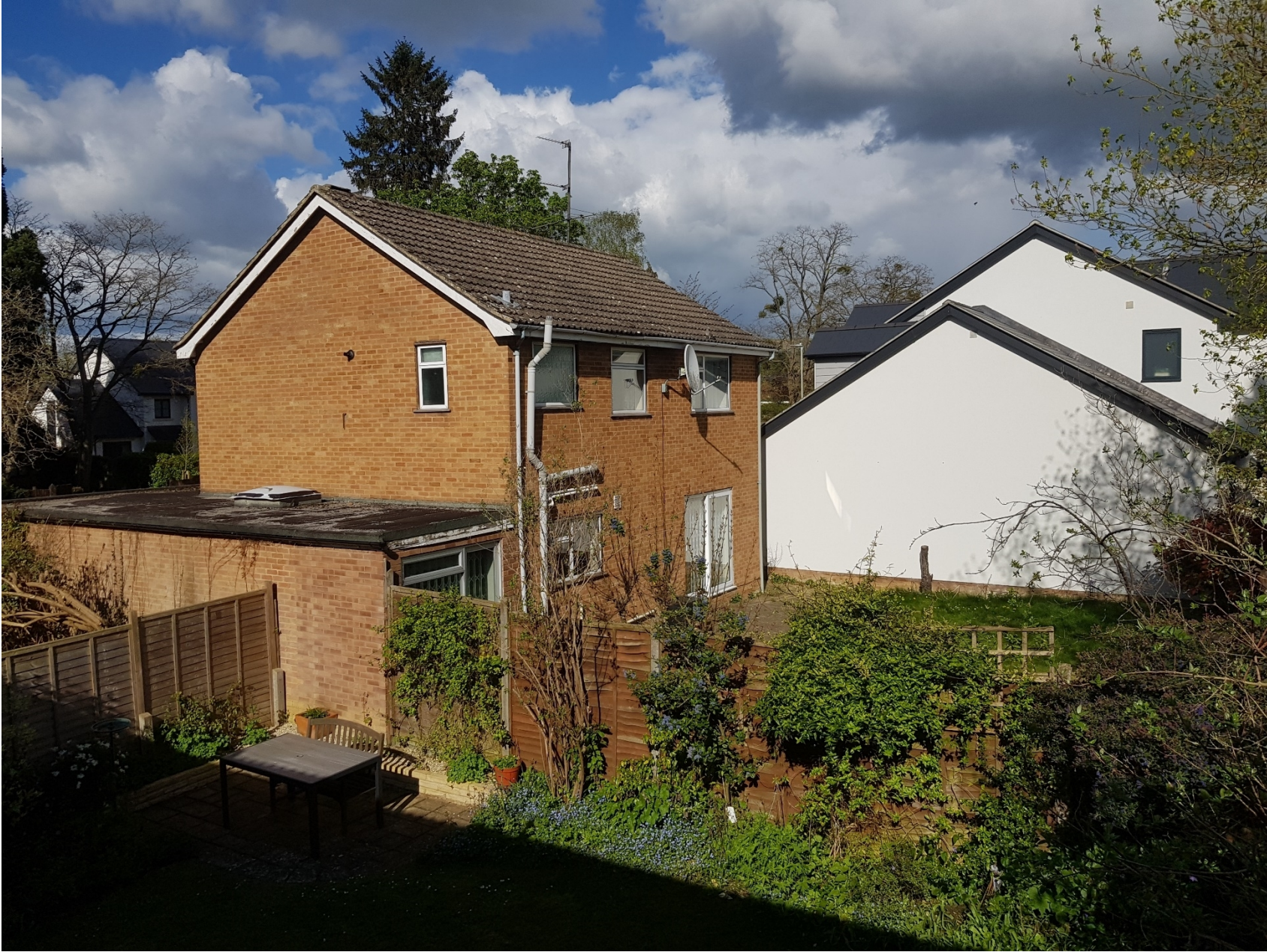
Photo of the application site from rear bedroom window of number 2 The Gardens
